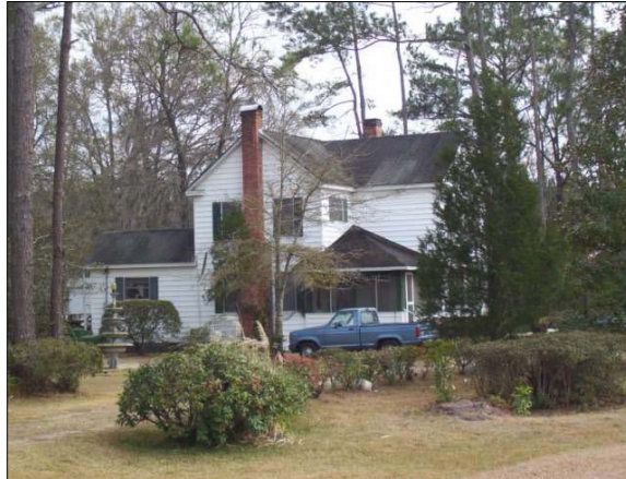
Figure 20, Braxton House, 1117 Steel Bridge Road.
