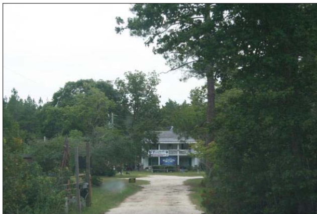
Figure 17, House at 64 Low Country Lane on the south side of Hwy 57/99.
